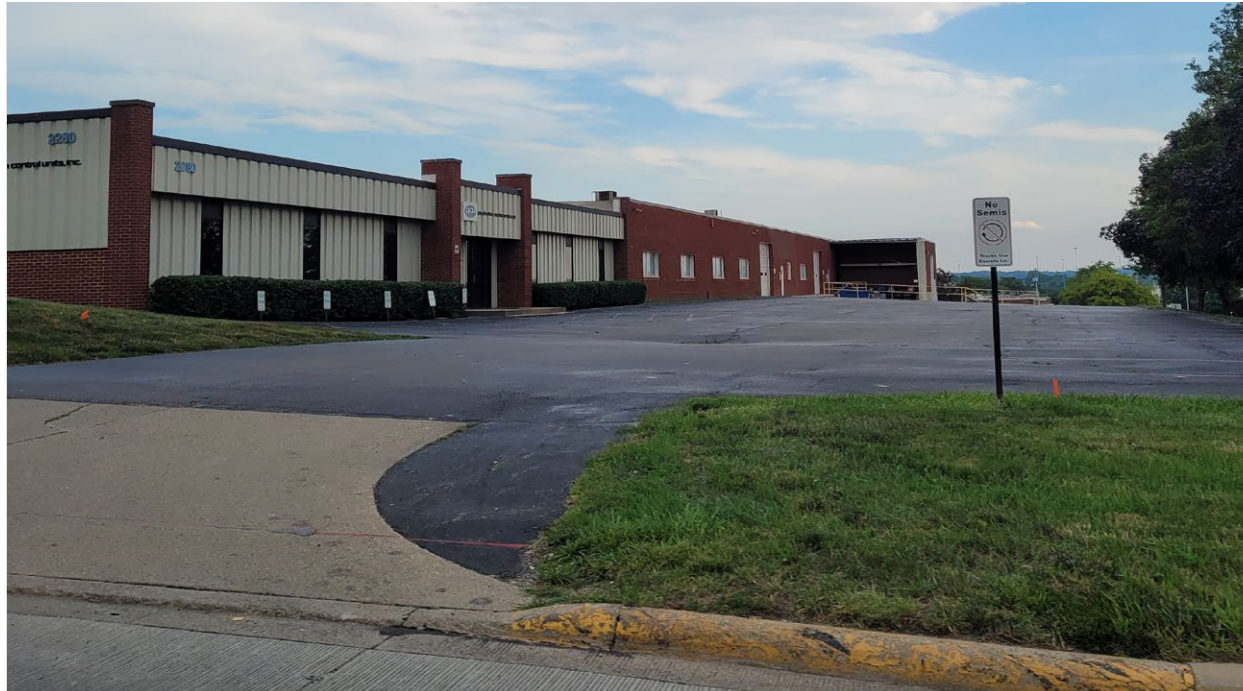
Fuyao is an example of the range and size of industrial activities permitted in an M-2 district. Source: American Structurepoint Inc.
